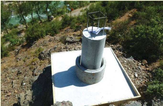
Pillar under construction
